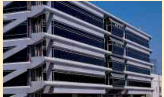
Adding bullnoses along each window ledge of the Terminal Services Building at the Hyperion Wastewater Treatment Facility added variety to the design, improved the proportions of the facade, and created changing light patterns during the day.
