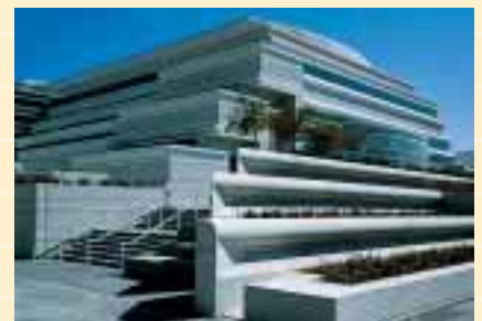
The lobby facade of the Moscone Convention Center makes ample use of bullnose sections, tying in with planters and adding visual interest to the center. (For another view of this project, see the Designer's Notebook cover, page 13.)
